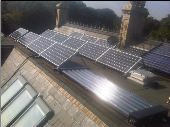
Half-way through the Solar Installation.
