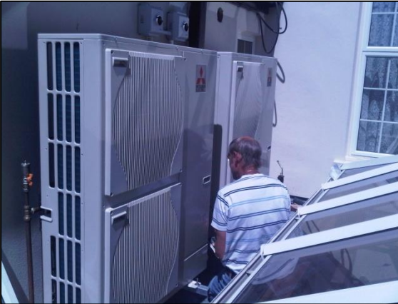
Art Installing the Heat Pumps.
