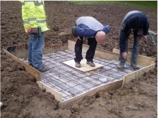
Project Engineer, Craig checks the Pit.
